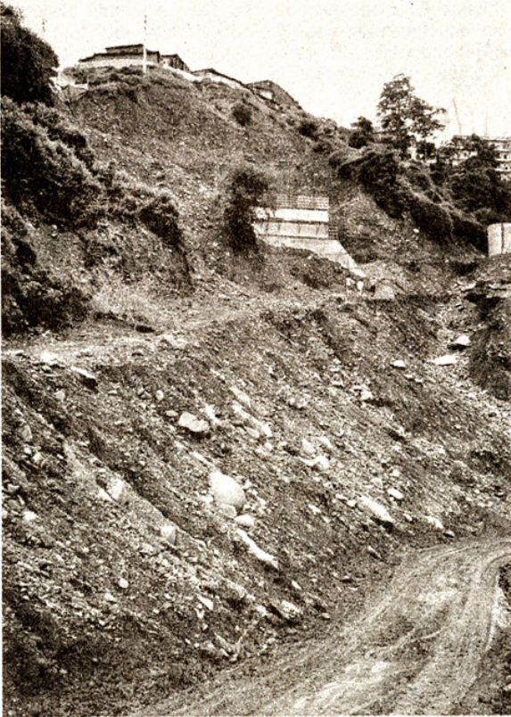
A view of the ecological degradation caused by construction of a by-pass road near Kamli at Parwanoo in Himachal Pradesh.
